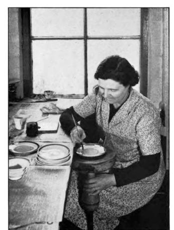
Banding and Gilding is done on the wheel which is revolved as desired by the operative's left hand. The accuracy and skill of Shelley Banders is astonishing
