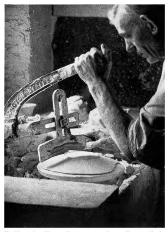
The Platemaker. Plates and saucers are made on a jigger upside down on a mould which shapes the upper surface or face of the article. A specially shaped tool which is pressed down by the operative, squeezes out the clay to the desired thickness, and shapes the back or underside
