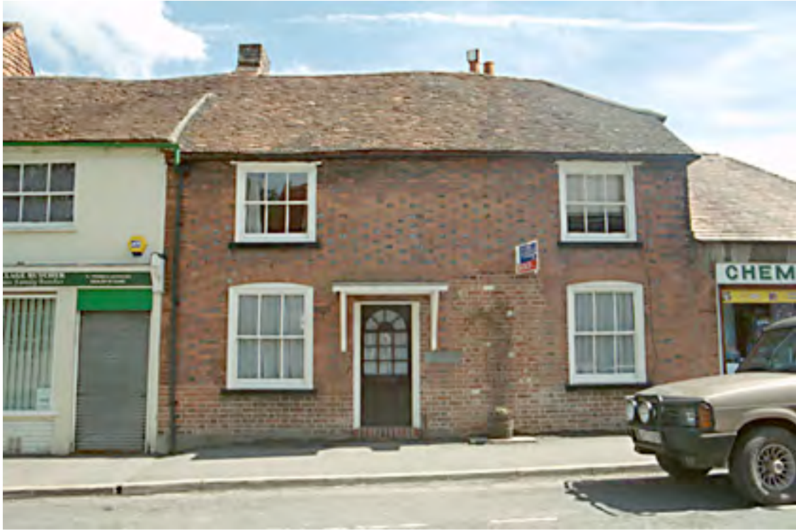
9 Swan Street, The Old Blacksmiths House
