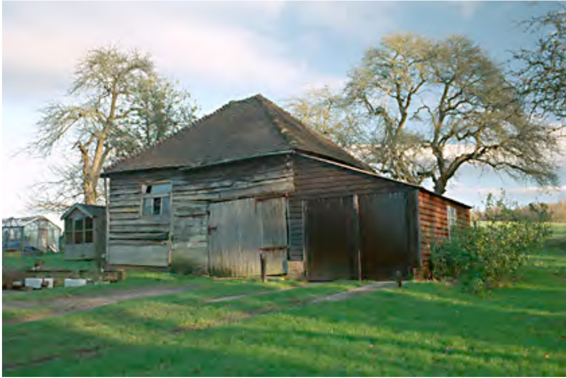
Small barn or granary at Harriden Farmhouse, Union Lane
