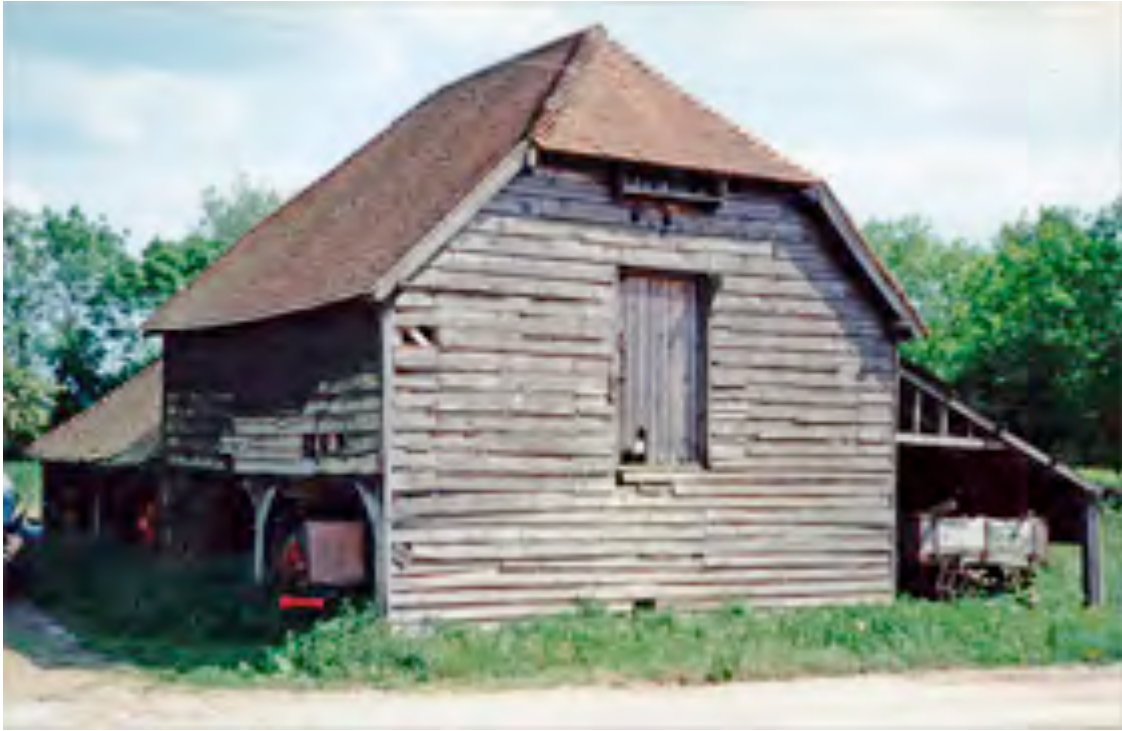
barn at Coldridges Farmhouse, Newbury Road
