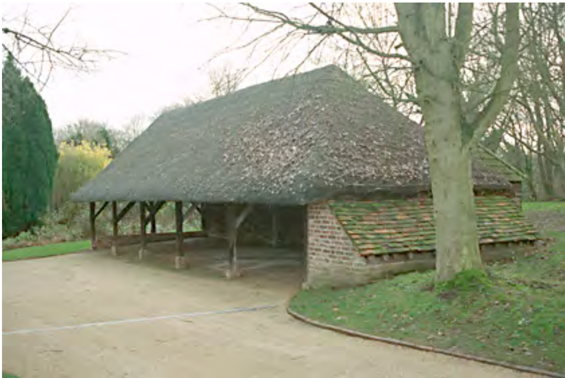
Cartshed at Island Millhouse, Union Lane
