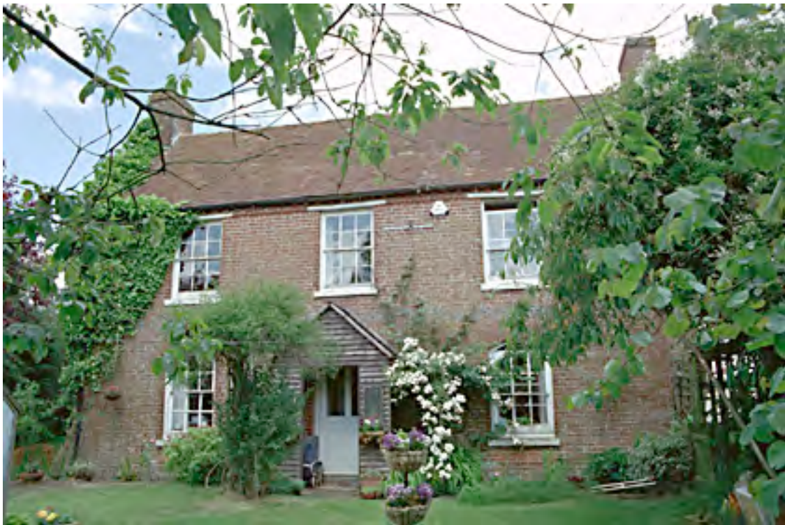
Coldridges Farmhouse, Newbury Road
